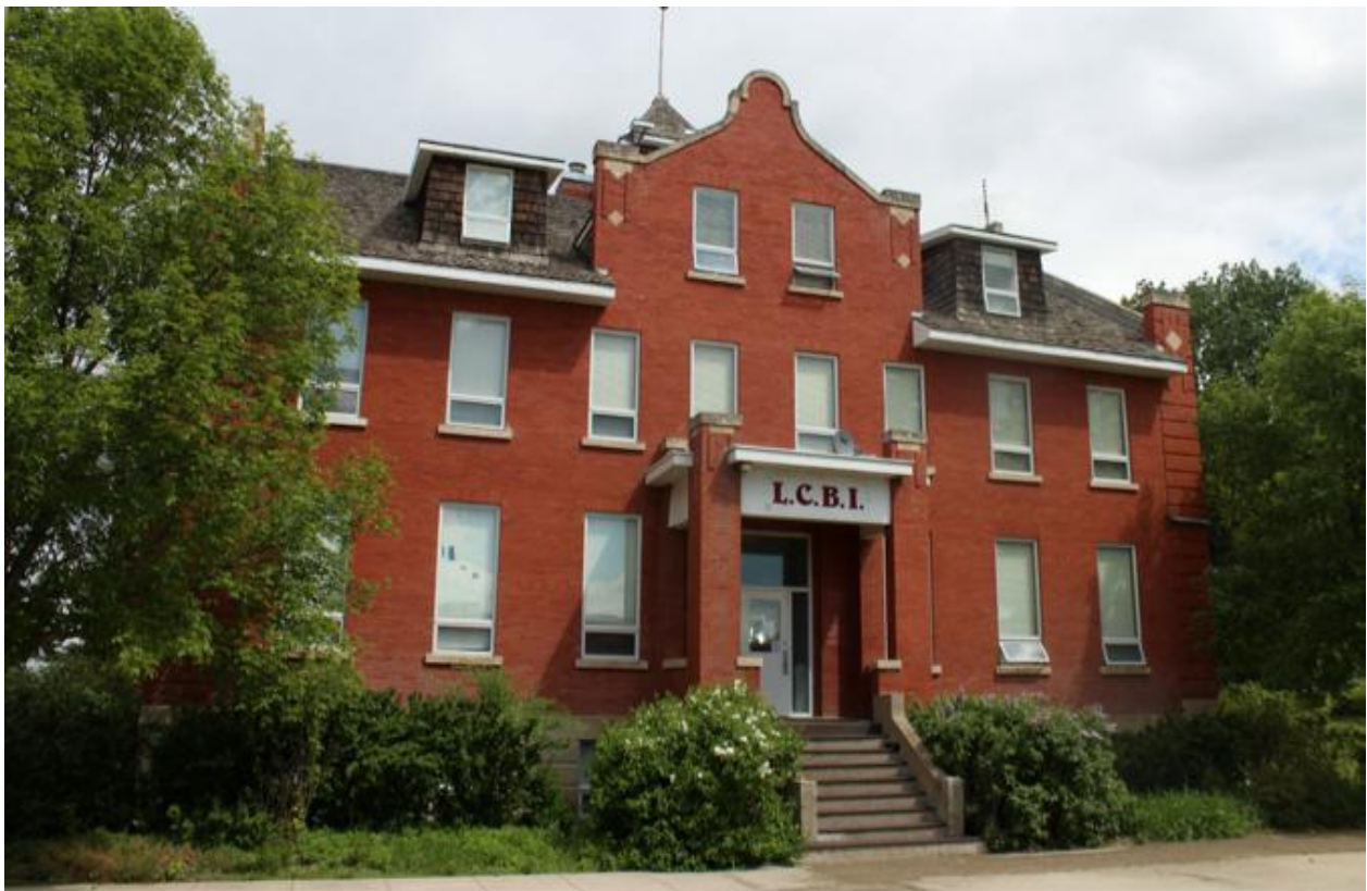
Old Main, the original building of OC / SLBI / LCBI, dedicated in July 1916
