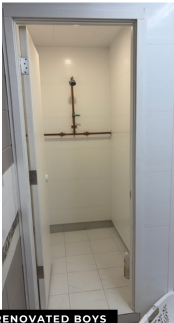
RENOVATED BOYS DORM SHOWERS
